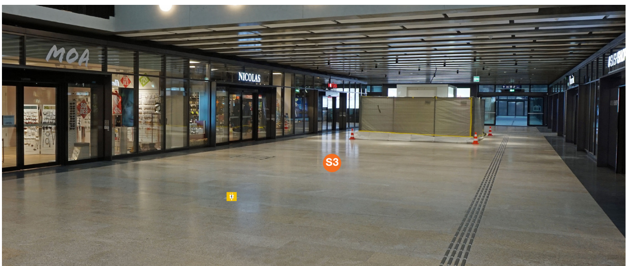
S3 Distribution point, Genève Eaux-Vives - Galerie Commercial, retail floor, city level, between Nicolas, Fleuriot, Sushishop and MOA
