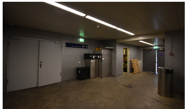
From the ramp, you can reach the P2 promotion area through an intermediate space.
