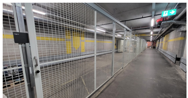
Logistics warehouse. 'Lager 3'. There is a power connection in the storage room.
