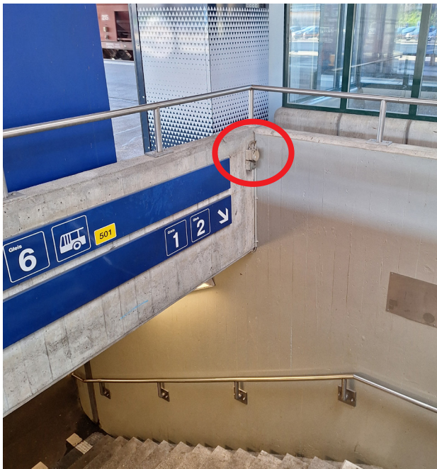
Power connection 230V 13A
